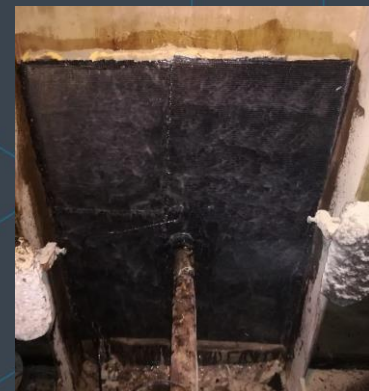
APPLICATION OF CARBON FIBRES
