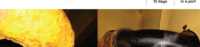
500m of ballast piping was heavily corroded and it was leaking sea water on numerous places. Minding all the safety standards, the repair lasted 12 days and it was conducted during the vessel's dry docking.
